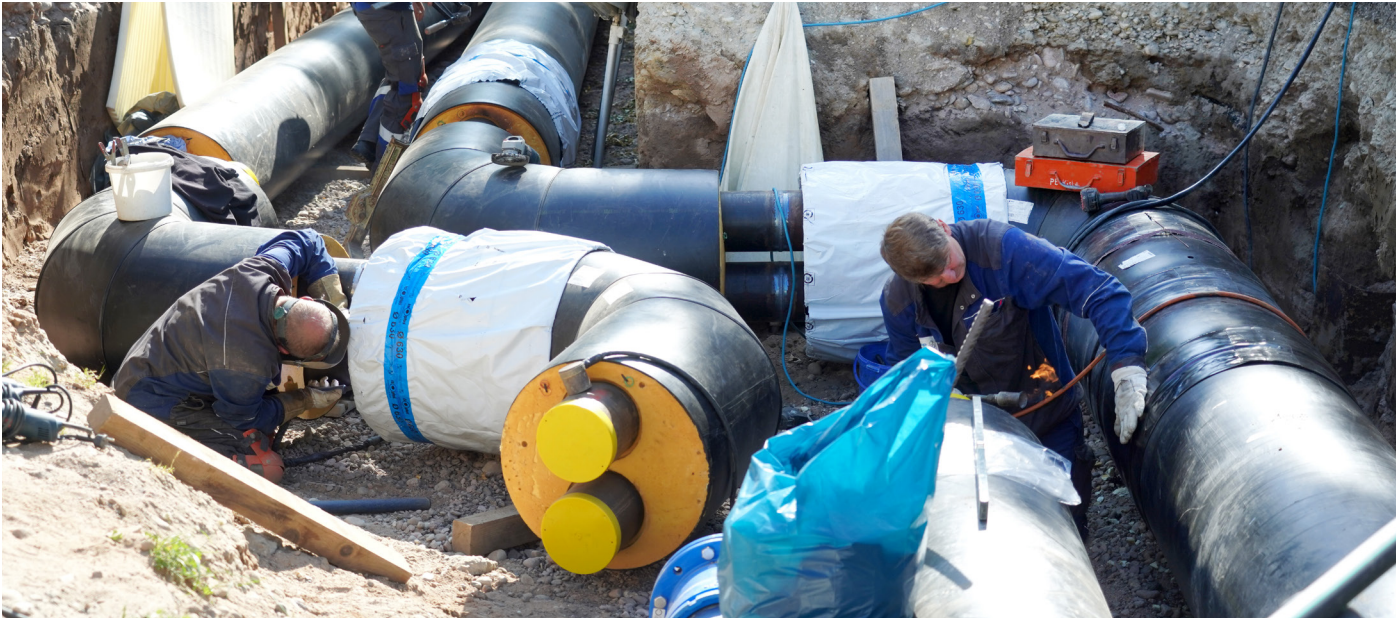
KEA-BW Agency supports municipalities in various ways, including heat planning and local heating network construction
