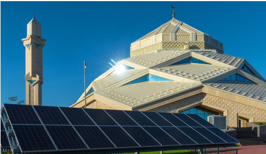
The Yrskeldi Qazhy Mosque in Kazakhtan's capital Astana is almost energy self-sufficient
